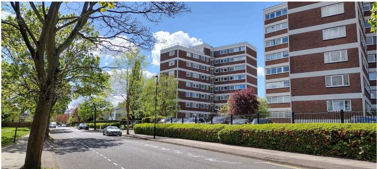
The two blocks of High Sheldon looking towards 63, 65 and 67 Sheldon Avenue
