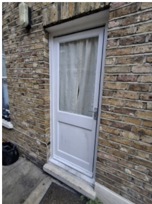
Rear Side Exit Door
