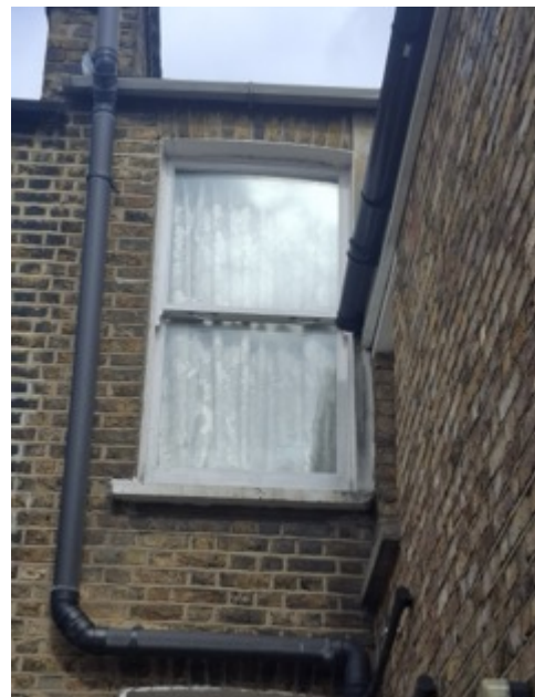
Rear Ground Floor Window
