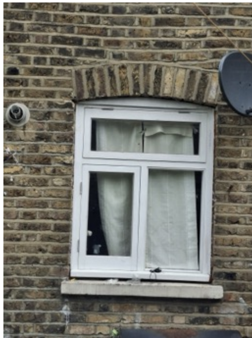
Rear End Ground Floor Window
