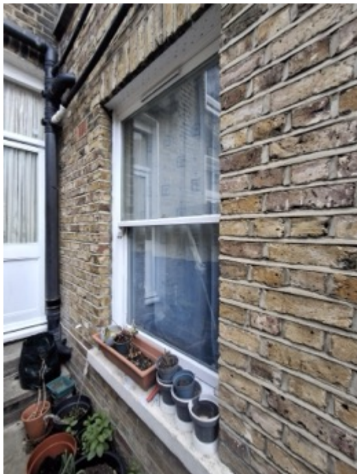
Rear Side Ground Floor Window
