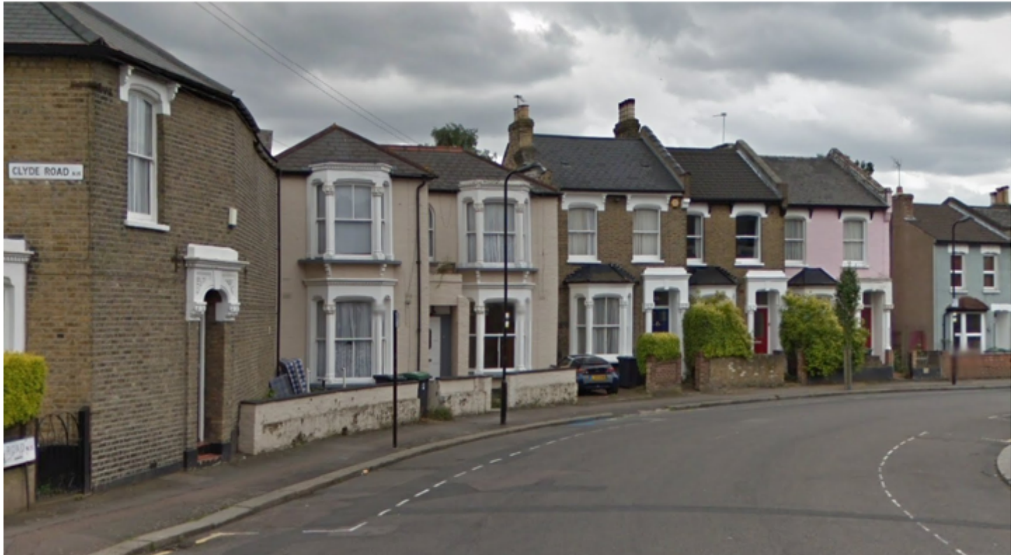
Google Maps 'Street View' of Clyde Road, Haringey, London, N15 4LS.
