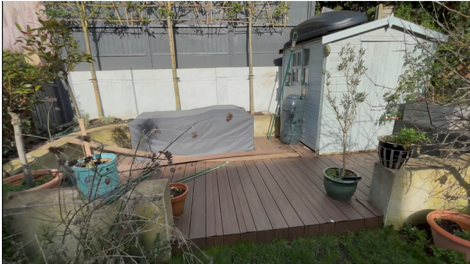
Existing Garden room / Retaining wall / decking
