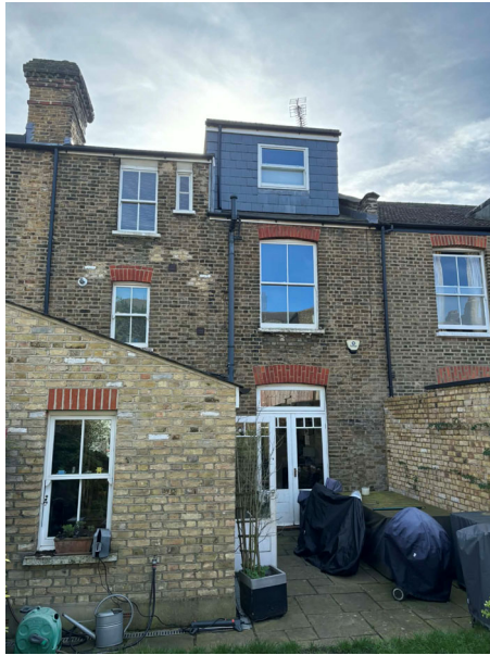
Existing Dormer and Extension
