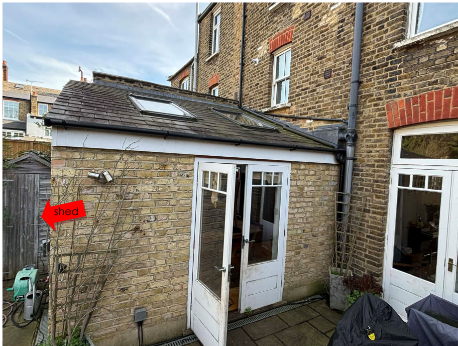
Existing Extension and tall garden shed/fence
