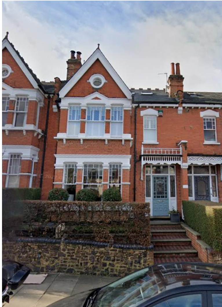
View of application site
