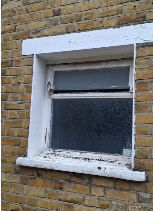
Rear End Ground Floor Window
