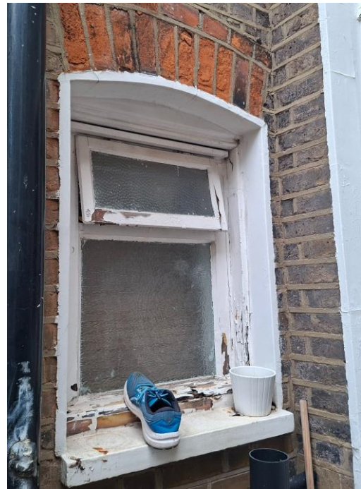
Rear Side Ground Floor Window
