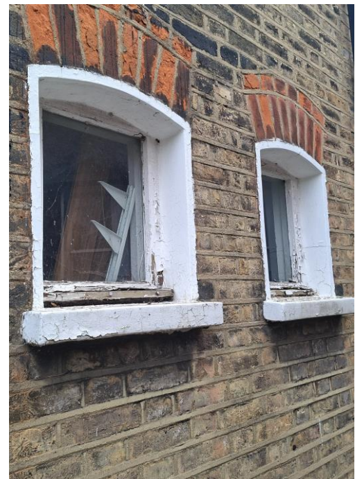
Rear Side Ground Floor Windows
