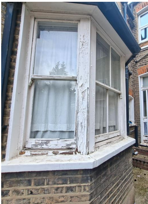
Rear Side Ground Floor Bay Window
