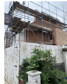
Looking towards 23, Forfar Road (side extension under construction)
