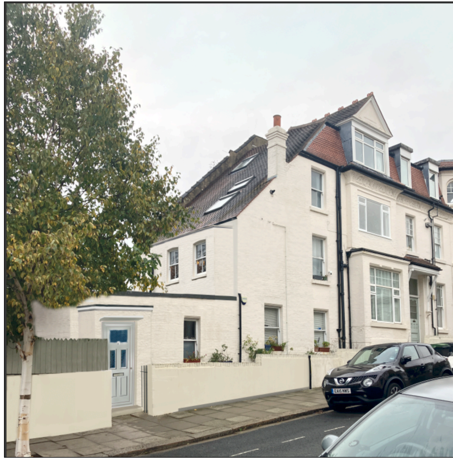
Existing rear side of No 11 from Milton Avenue - note existing entrance via the private garden
