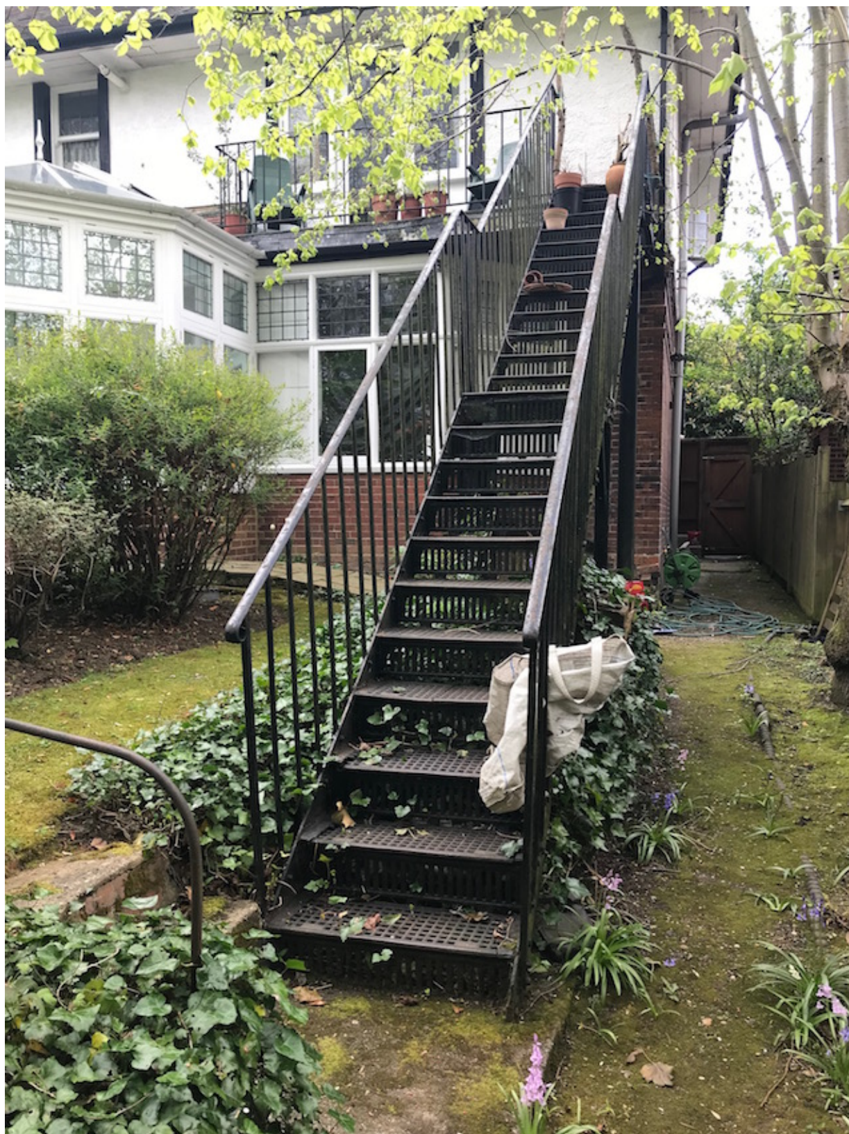
View from the rear garden showing the metal staircase and balcony (to be removed), side access path and boundary with no.31 on the right
