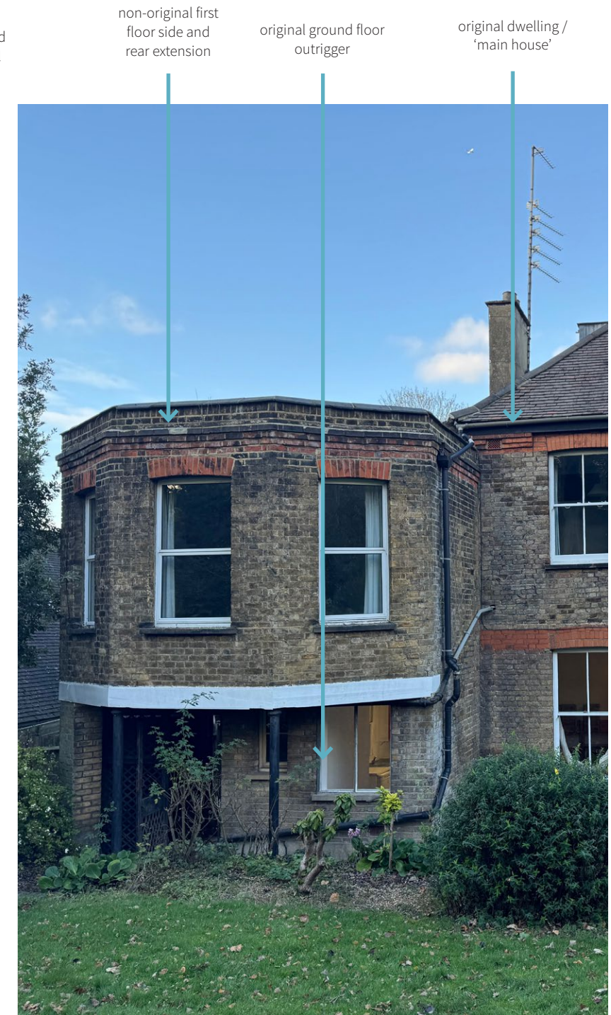
Mid 20th Century rear extension
