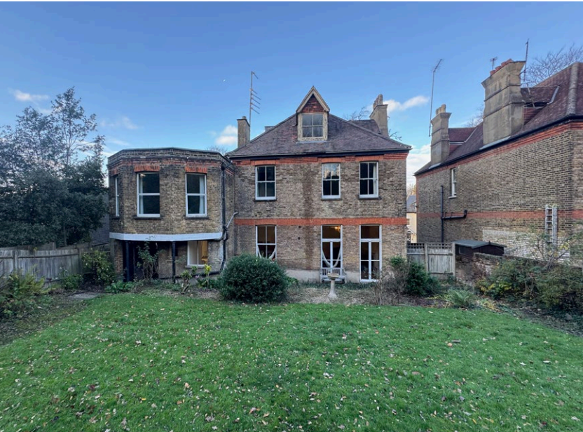
The existing rear elevation and garden
