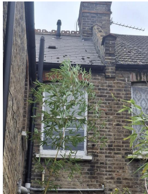
Rear First Floor Window
