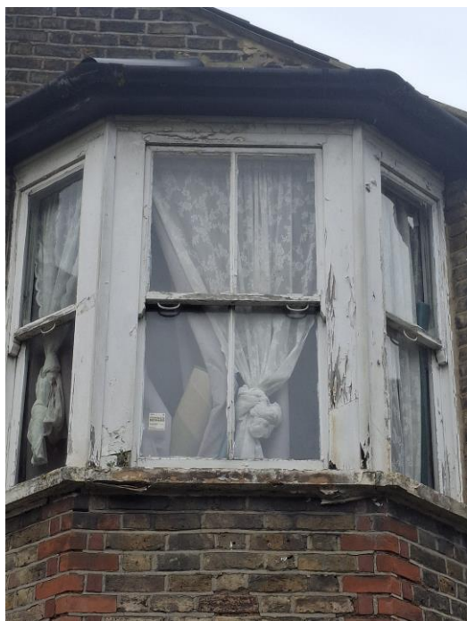
Rear End First Floor Bay Window
