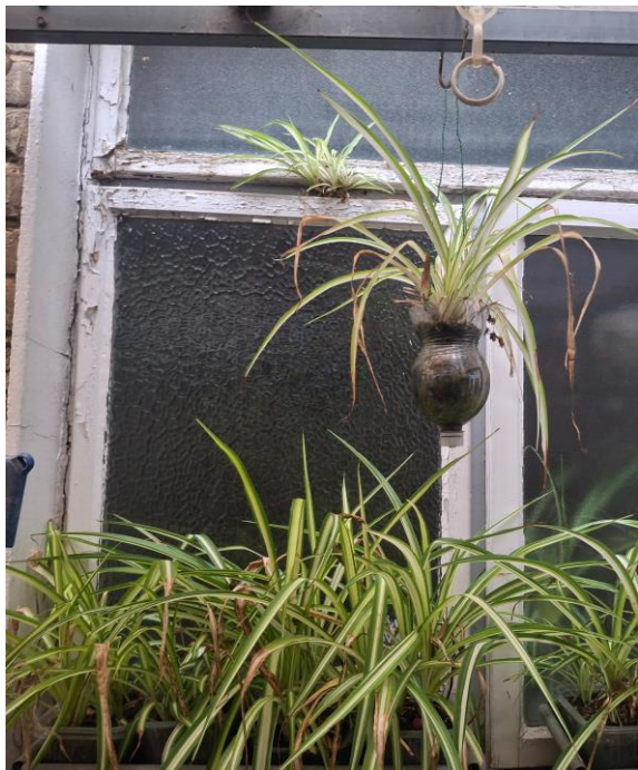
Rear Side Ground Floor Window
