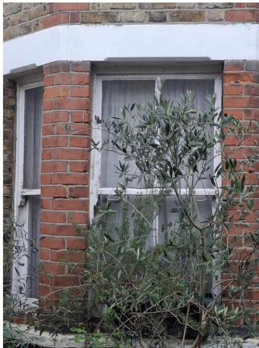
Rear End Ground Floor Bay Window
