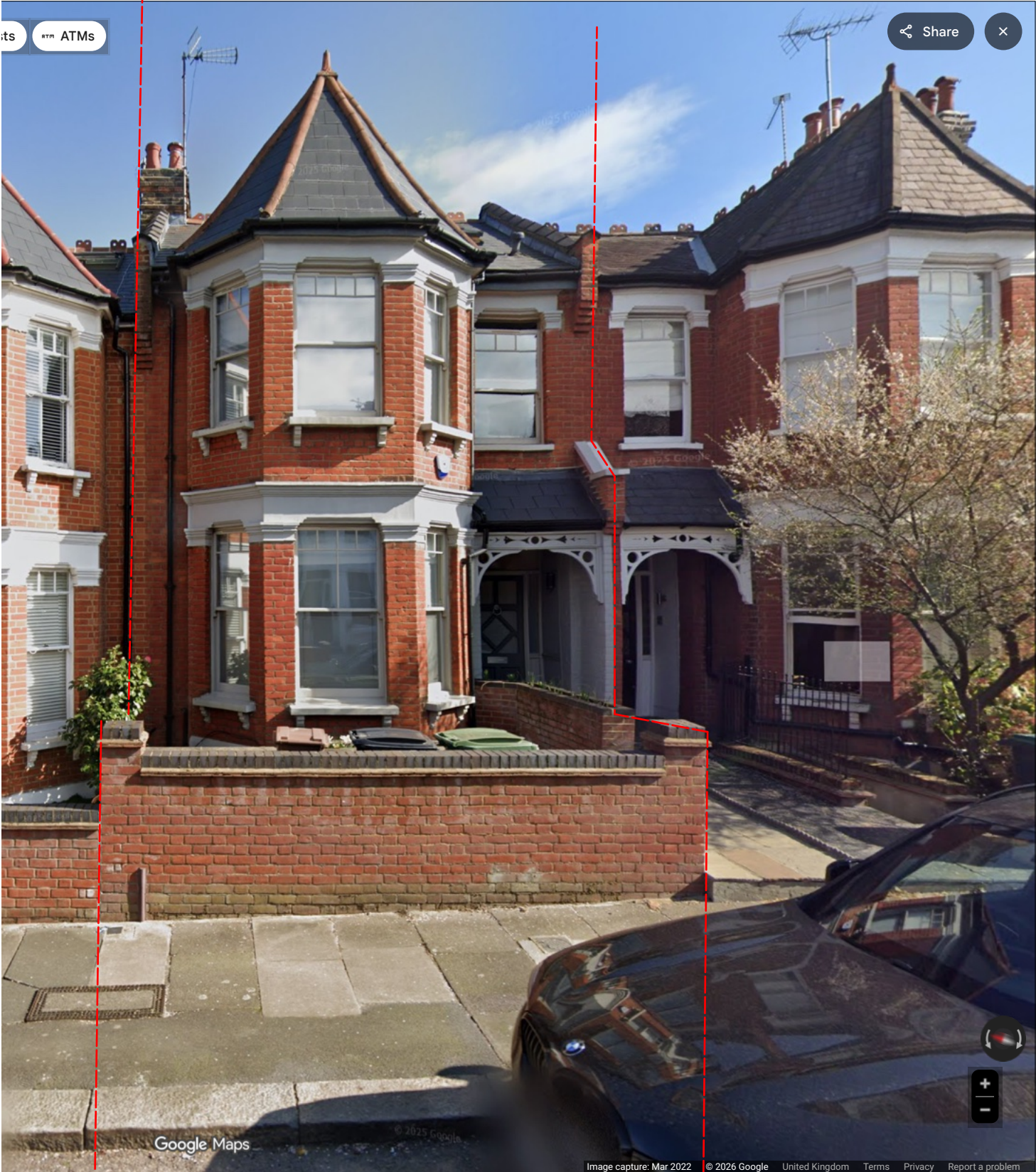
APPLICATION SITE FRONT ELEVATION PHOTOGRAPH
