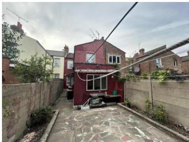
Fig. 1 — Rear elevation showing the existing 1990s kitchen extension whose building line will be retained.
