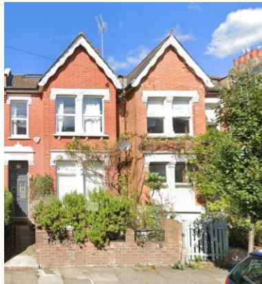
Fig. 5 — Original red brickwork on the opposite side of Sirdar Road, illustrating the tone proposed for the side-return infill.
