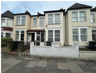
Fig. 1 — Front elevation of No. 22, showing the later cement render obscuring the original brickwork.
