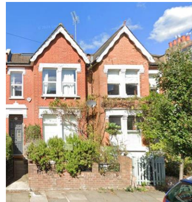
Fig. 3 — Properties opposite retaining original brickwork, illustrating the intended appearance of the front facade following render removal.
