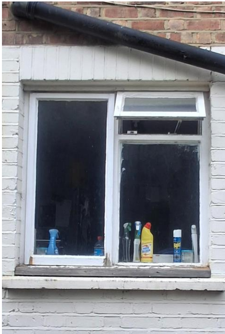
Rear End Ground Floor Window
