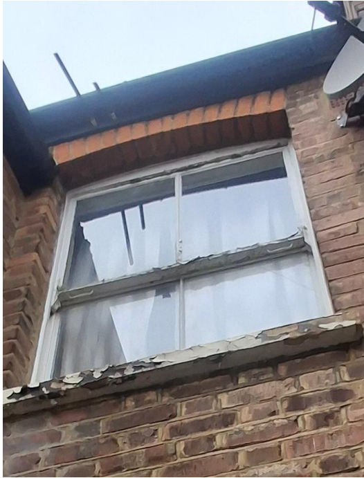
Rear First Floor Window
