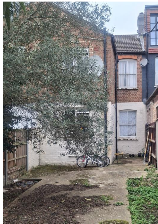
Rear Side Elevation (South East)
