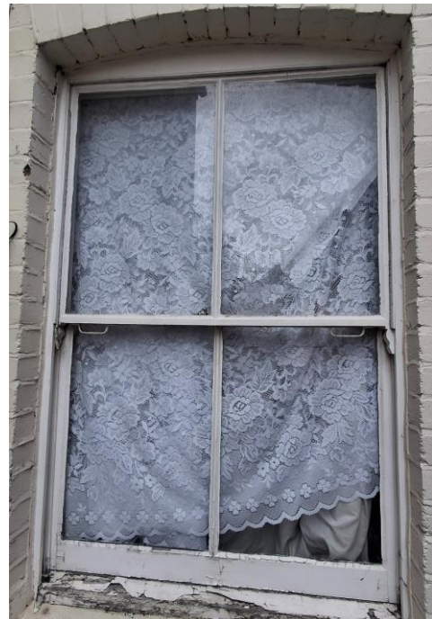
Rear Ground Floor Window
