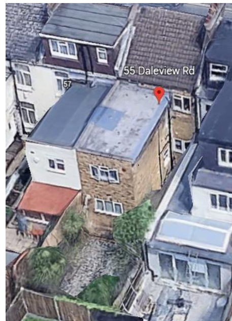
Rear Elevation View (no images available)
