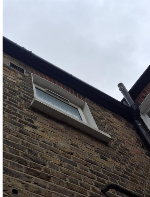
Rear Side First Floor Window
