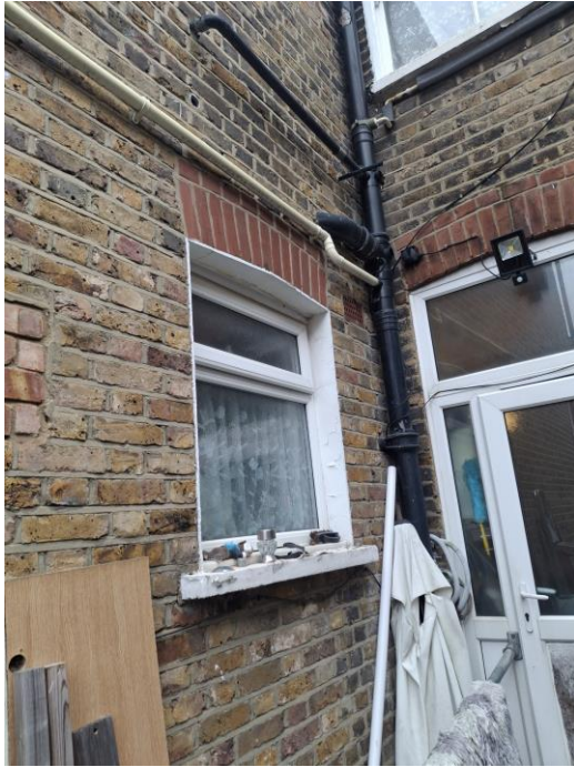
Rear Side Ground Floor Window
