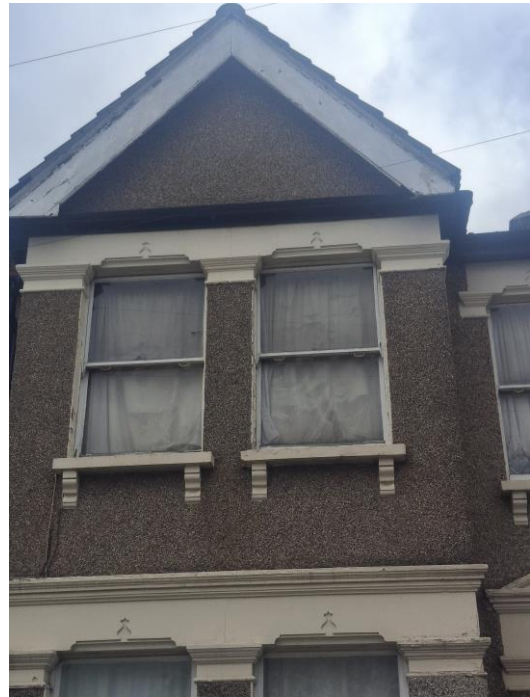
Front First Floor Windows
