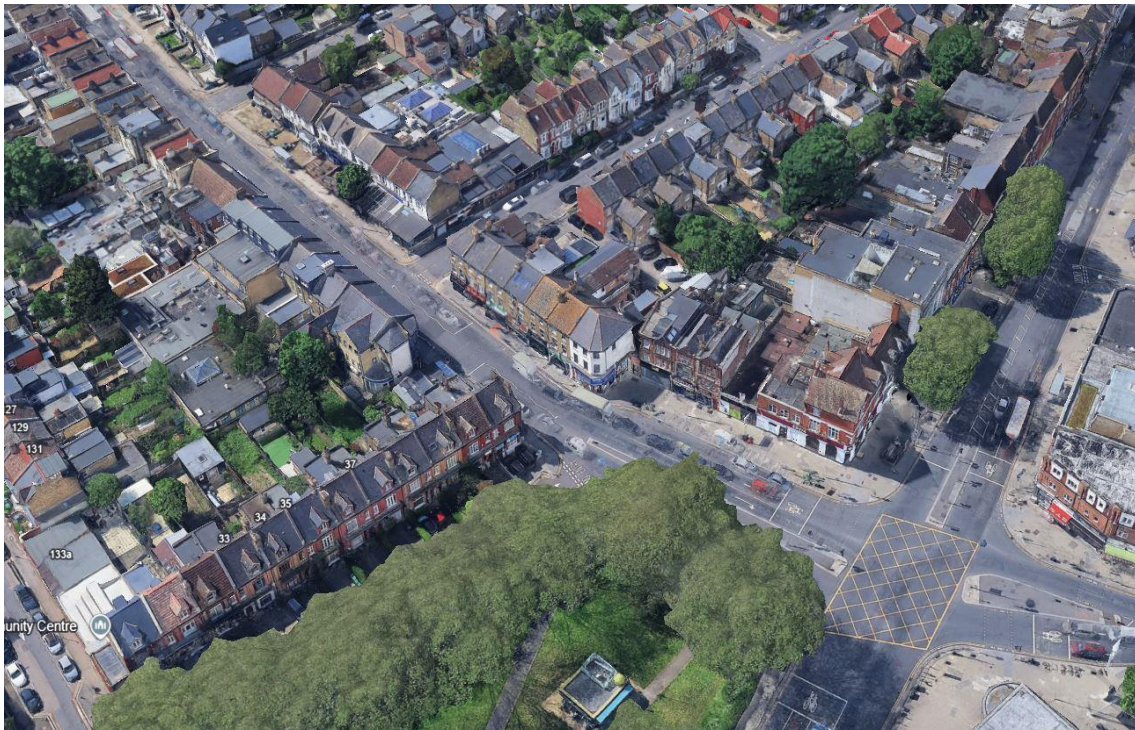
AERIAL VIEW OF SITE
