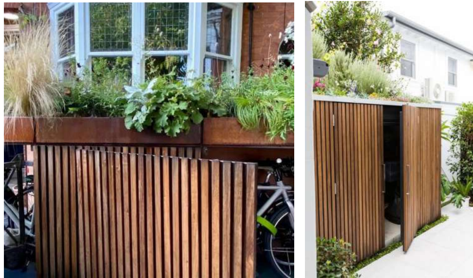
Timber cladding bike store with green roof
