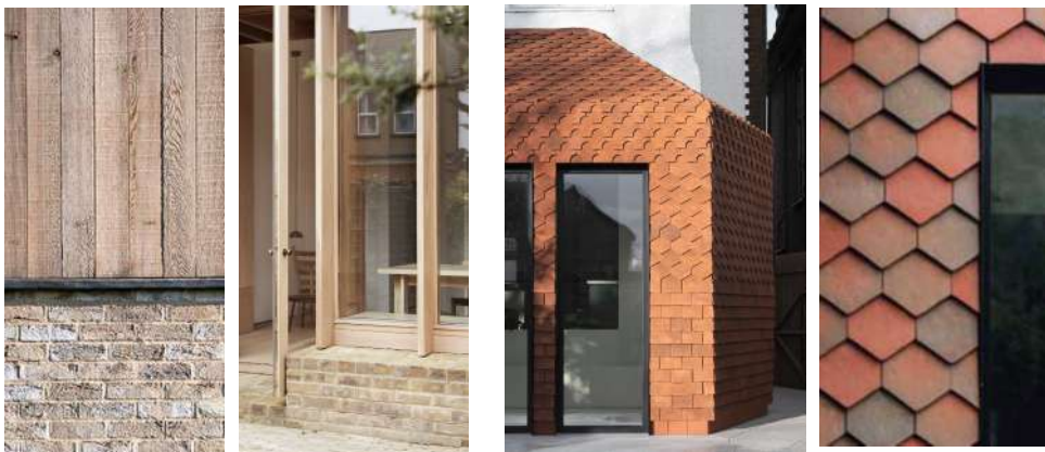
Brick base with timber cladding above
