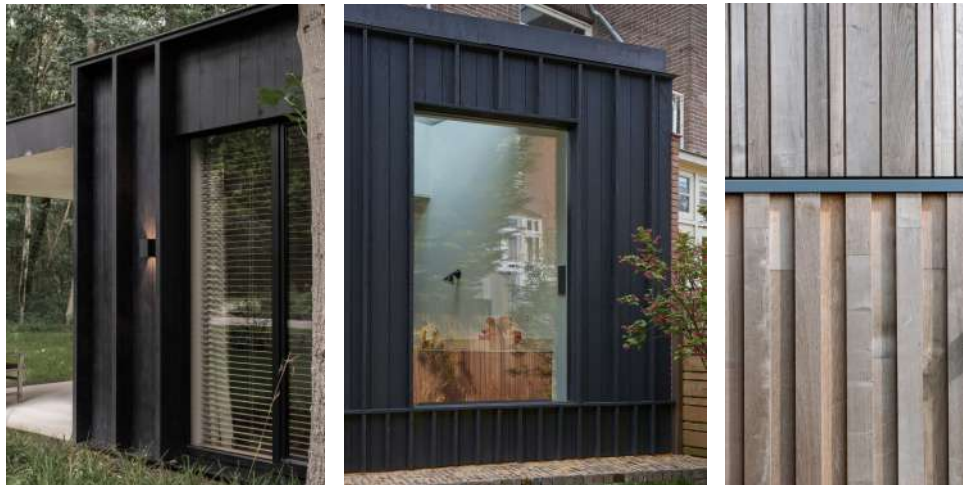
Timber cladding and vertical timber fins
