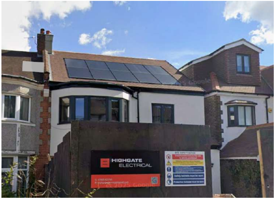
EWI and solar panels at no.7 Wood Vale
