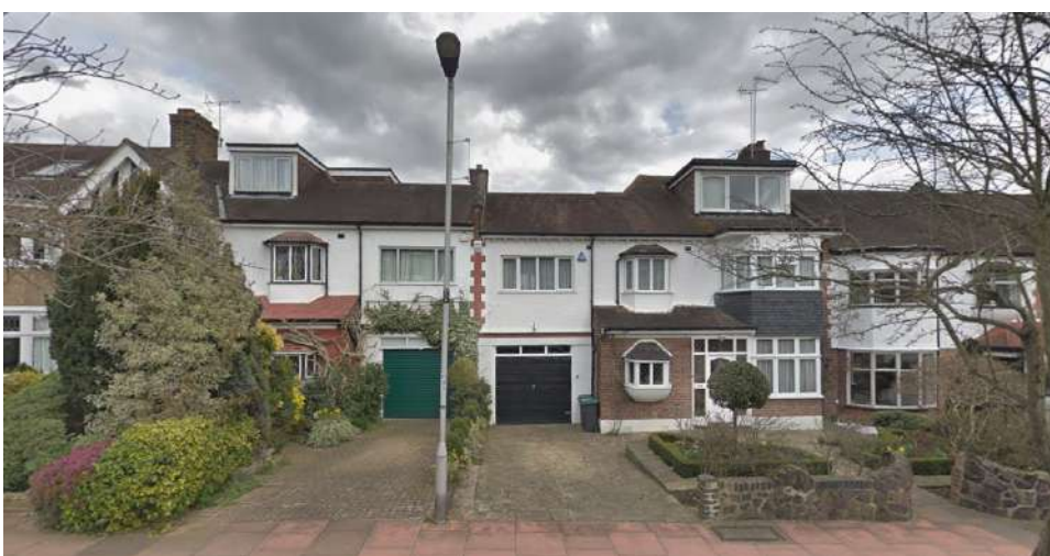
No. 27 & No. 29 Wood Vale, opposite the application site. Image from Google street view 2015
