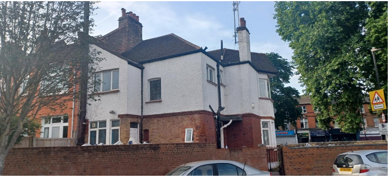
Photo 2: Side elevation / rear corner view from Rectory Gardens
