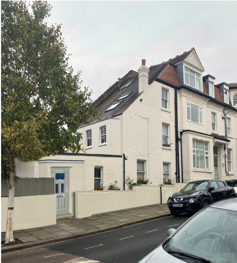
Existing rear side of No 11 from Milton Avenue - note existing entrance via the private garden
