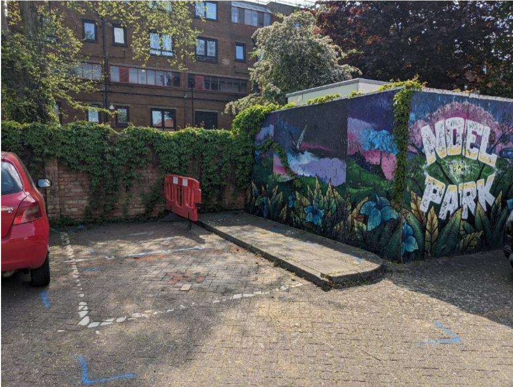
PHOTOGRAPH 3: WS101 BACKFILLED AND RE-INSTATED
