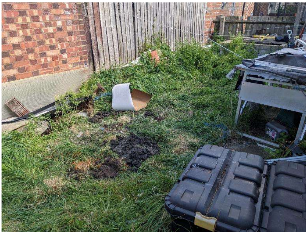
PHOTOGRAPH 13: HP104 BACKFILLED AND RE-INSTATED
