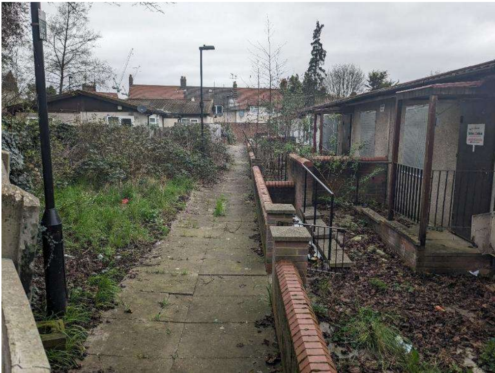
PHOTOGRAPH 3 – FOOTPATH ACCESS TO BUNGALOWS 1-5
