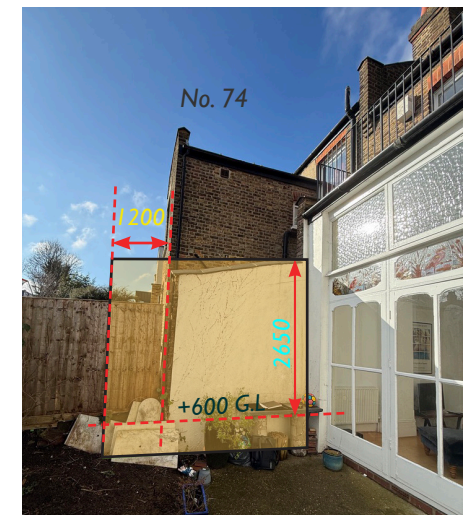
Fig 4.3- Photograph showing impact of extension on the boundary to no.74
