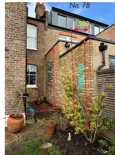
Fig 4.2- Photograph showing impact of extension on the boundary Approved Planning application HGY/2021/1539
