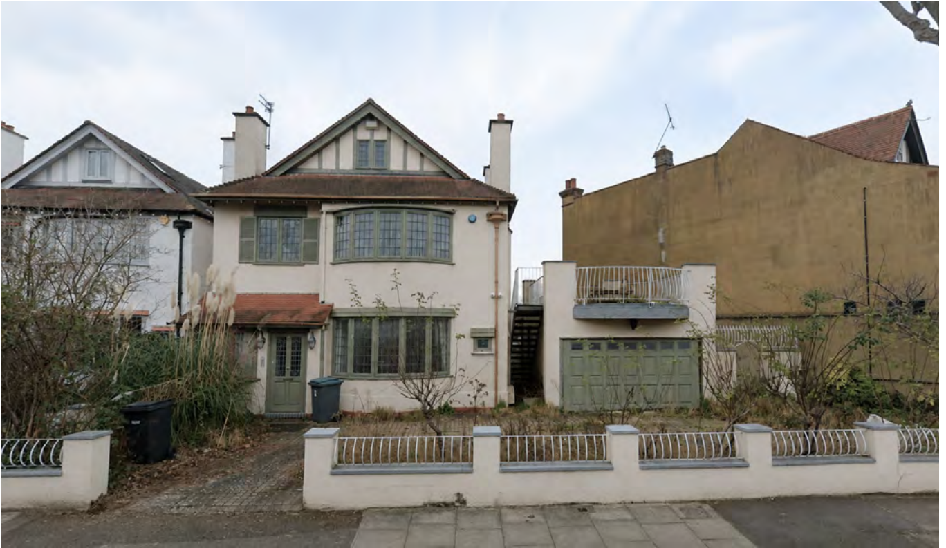
Existing house and boundary treatment
