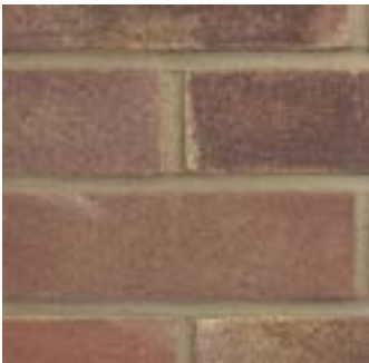
Running bond brickwork
