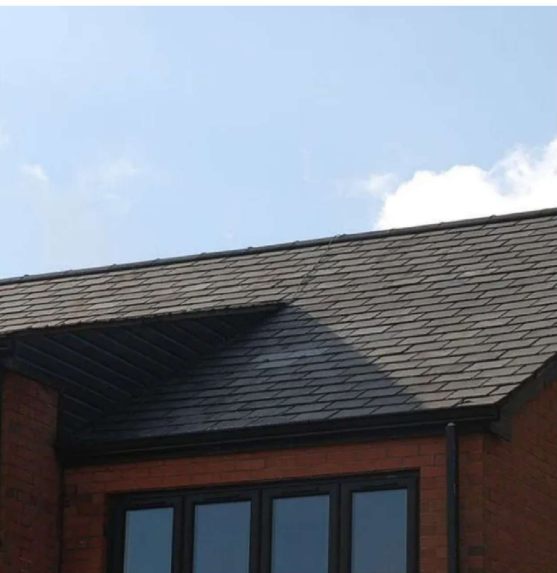
Passaro Natural Slate Roof Tiles to replace existing where necessary
