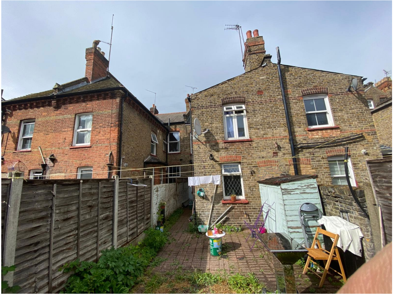
Rear Elevation Photo 2
