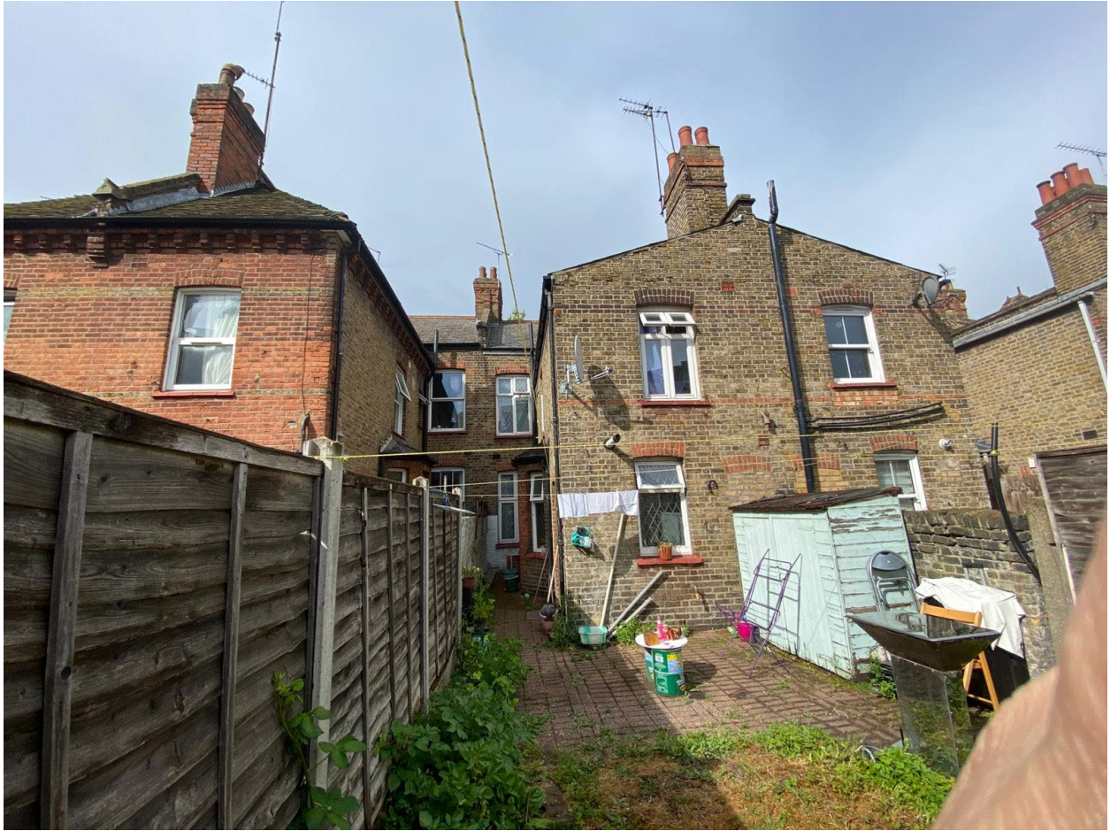
Rear Elevation Photo 1
