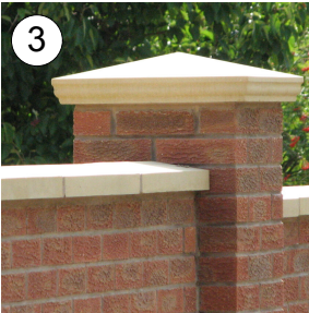
Brick wall and pillar with Yorkstone piers cap. Birtley Olde English Brick. Length: 28.1m
