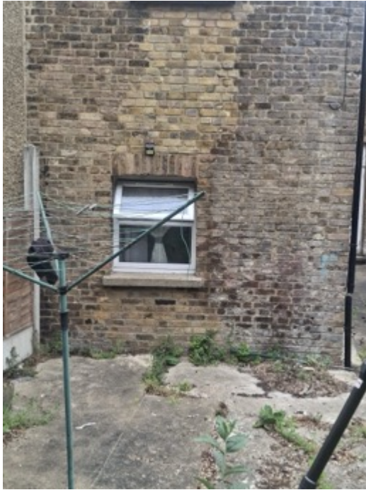
Rear End Ground Floor Window
