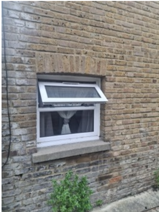
Rear Side Ground Floor Window
