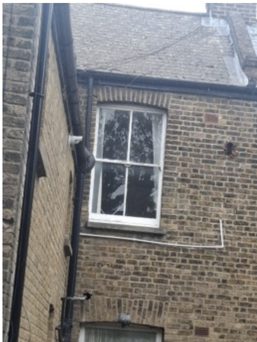
Rear First Floor Window
