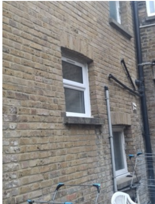
Rear Side Ground/First Floor Window
