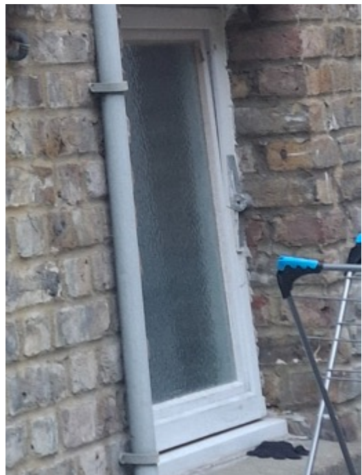
Rear Side Ground Floor Window
