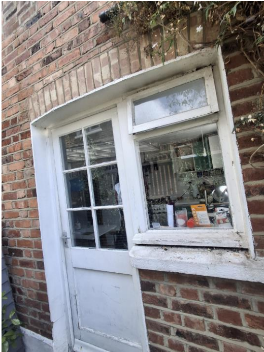
Rear Exit Door Ground Floor
