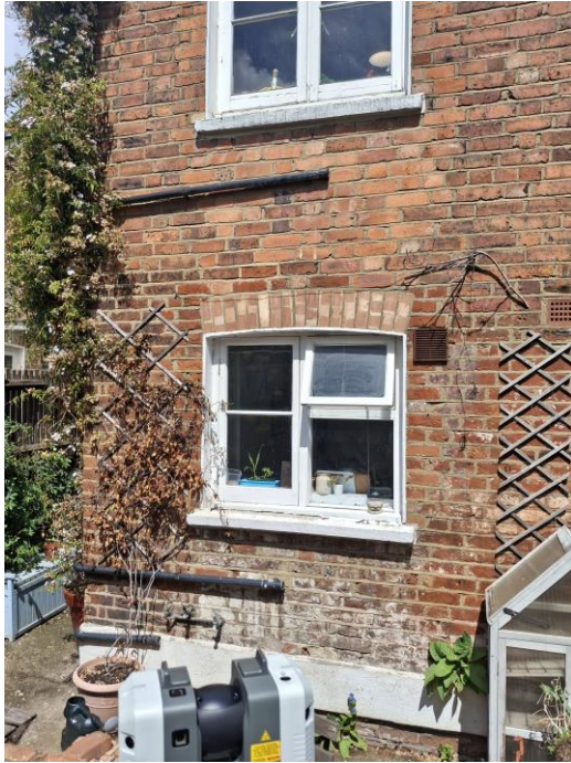
Rear End Ground Floor Window
