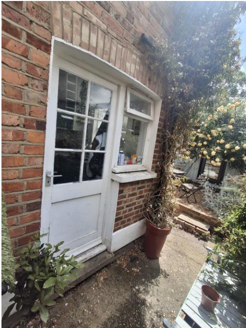
Rear Exit Door Ground Floor
