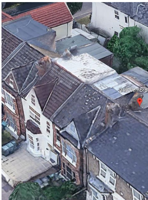
Roof Side Elevation (West)
