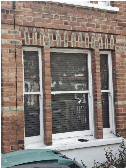
Front Ground Floor Window
