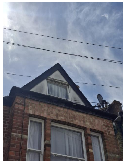
Front Second Floor Window
