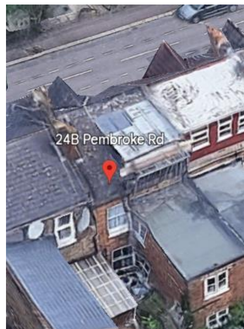
Roof Rear Elevation (South)
