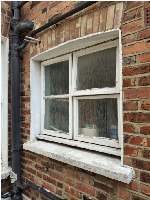
Rear Side Ground Floor Window
