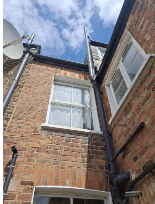
Rear First Floor Window
