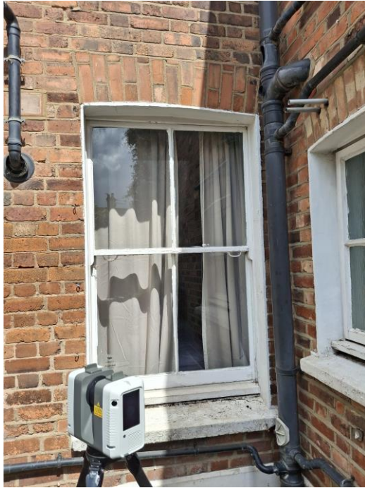
Rear Ground Floor Window
