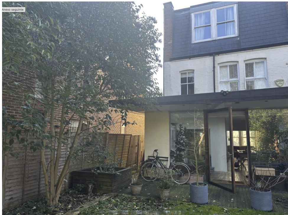
Image 3: Rear Façade – 4 Claremont Road
