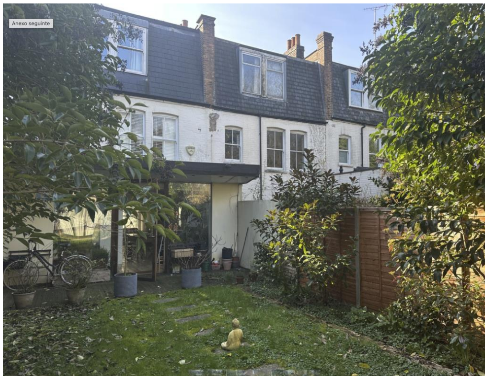
Image 4: Rear Façade – 7 Claremont Road
