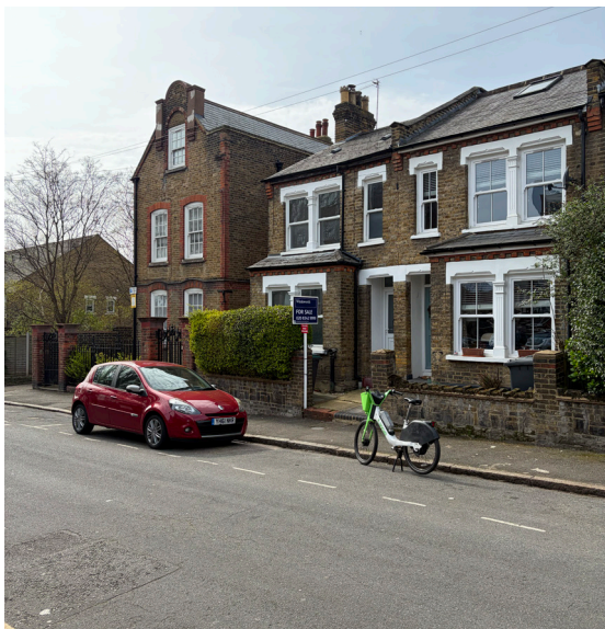
Figure 1: Photo of existing frontage
