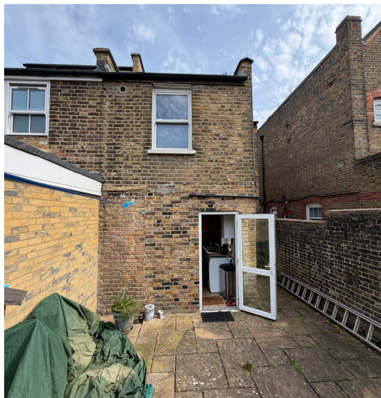
Figure 2: Photo of existing rear
