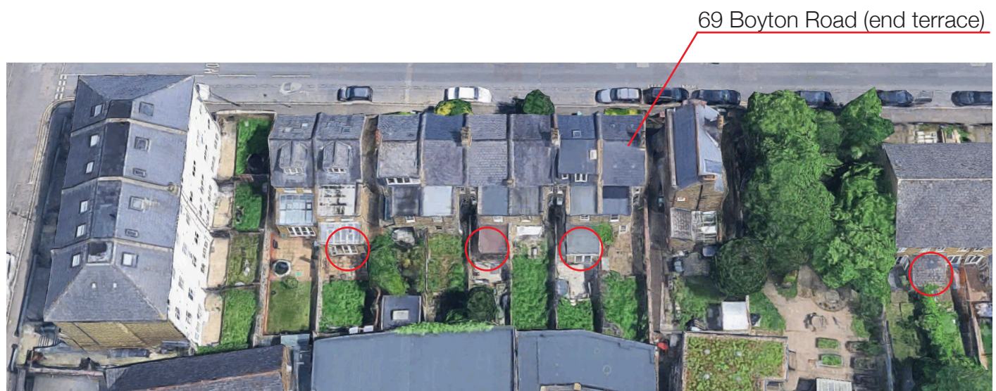
Figure 3: Existing rear-side extensions and alterations on Boyton Road highlighted with red circles.
