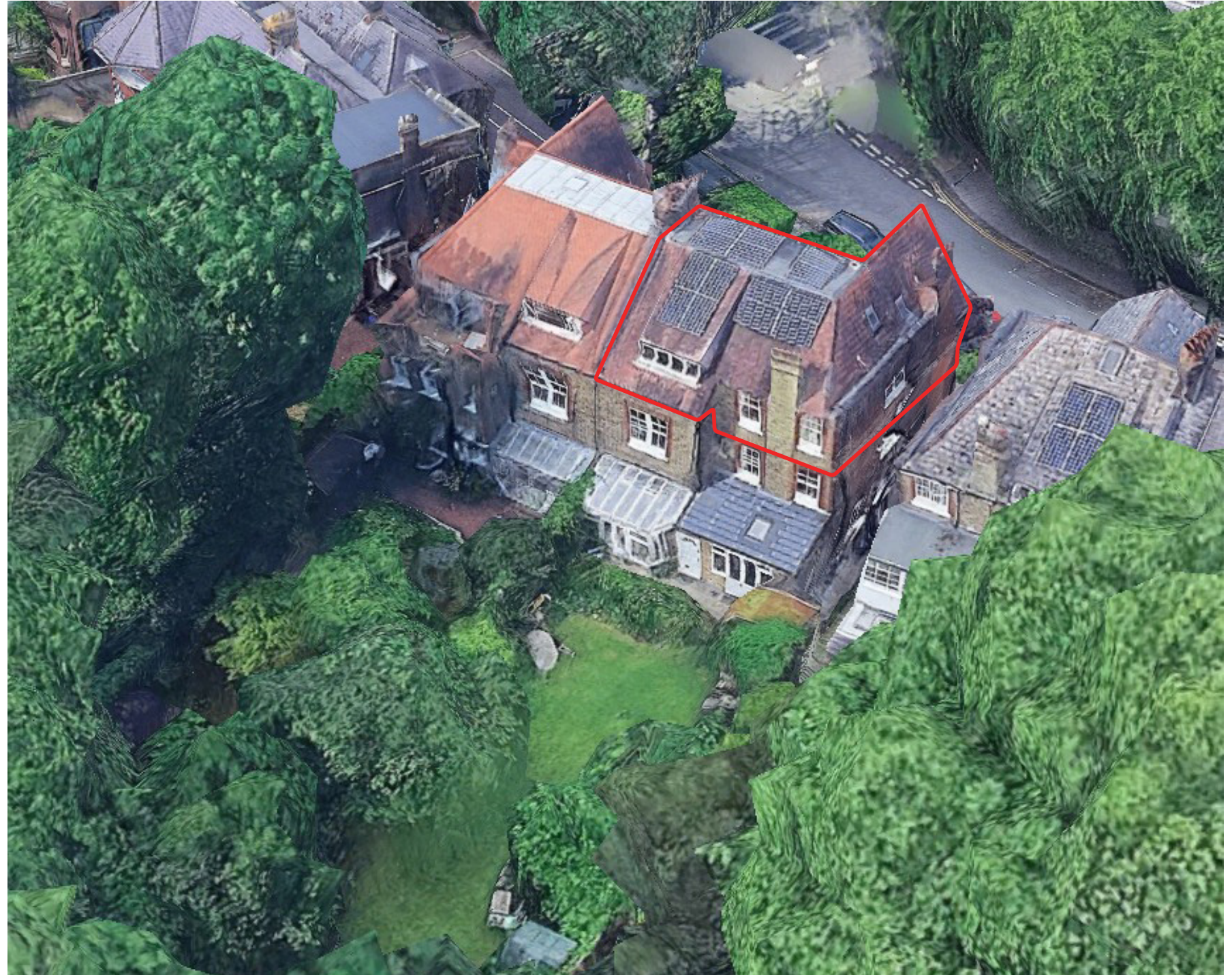
View of the rear of Haslemere Road, with No.8b outlined in red - Google Earth image
