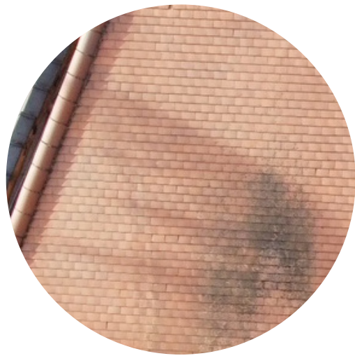
New tile cladding to gable to match the existing roof finish
