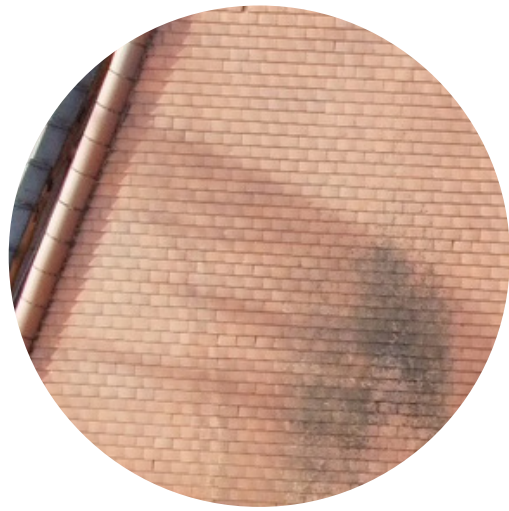
New roof tiles to match existing
