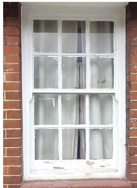
Rear First Floor Window
