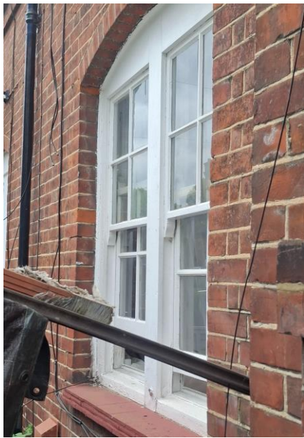
Front Ground Floor Window
