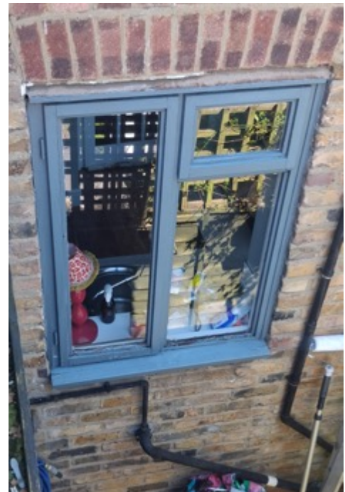
Rear Side Ground Floor Window
