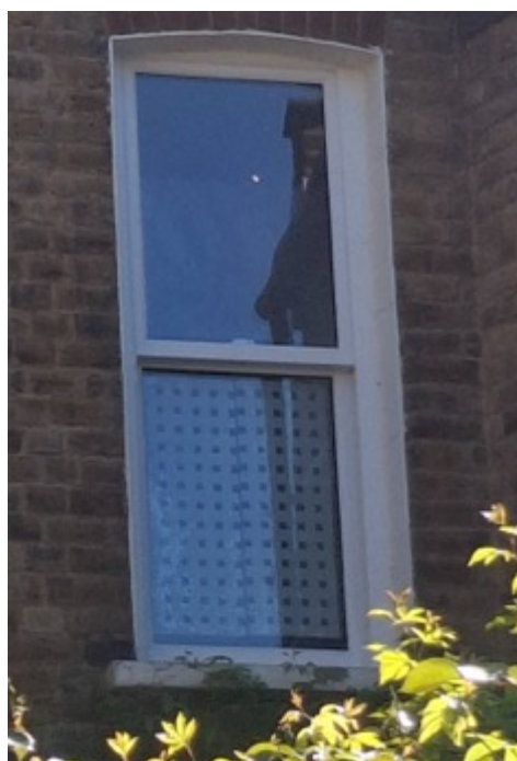
Rear First Floor Window
