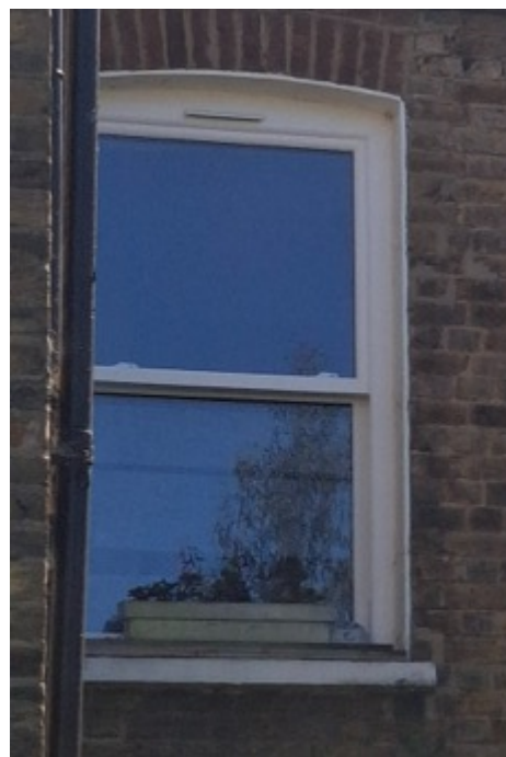
Rear First Floor Window
