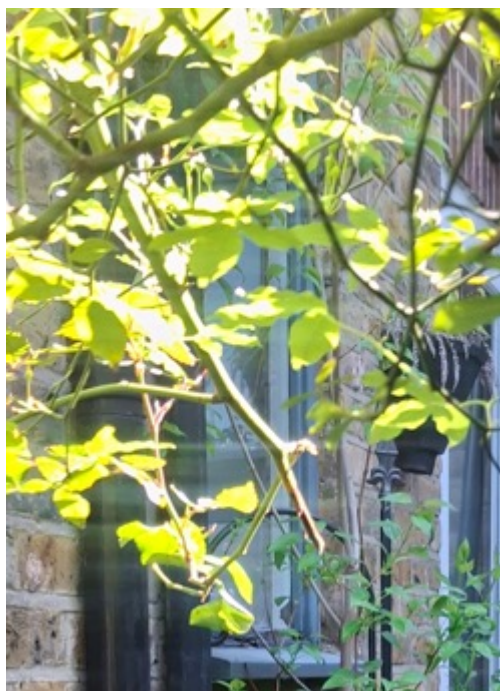
Rear Side Ground Floor Window
