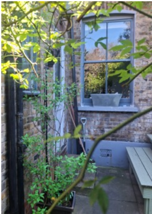
Rear Ground Floor Window
