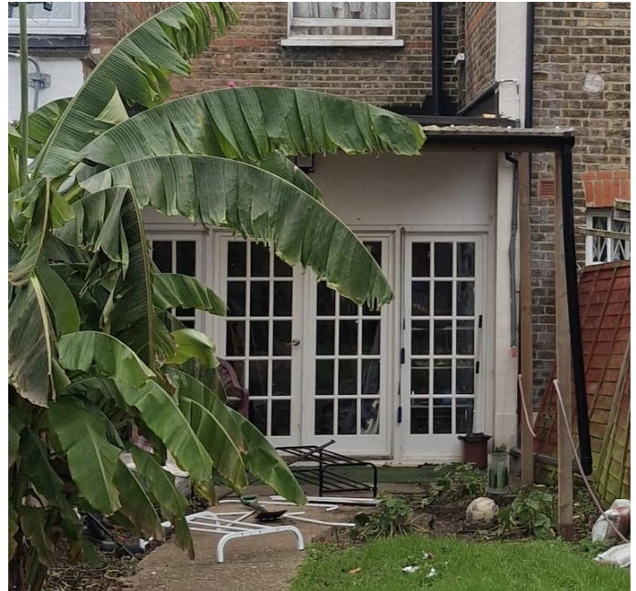
Rear Elevation Exit Door
