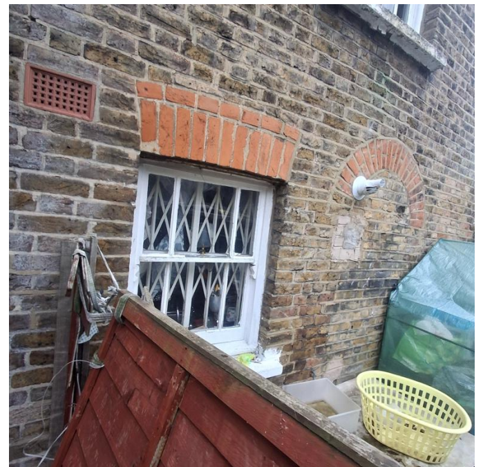
Rear Addition Ground Floor Sash window
