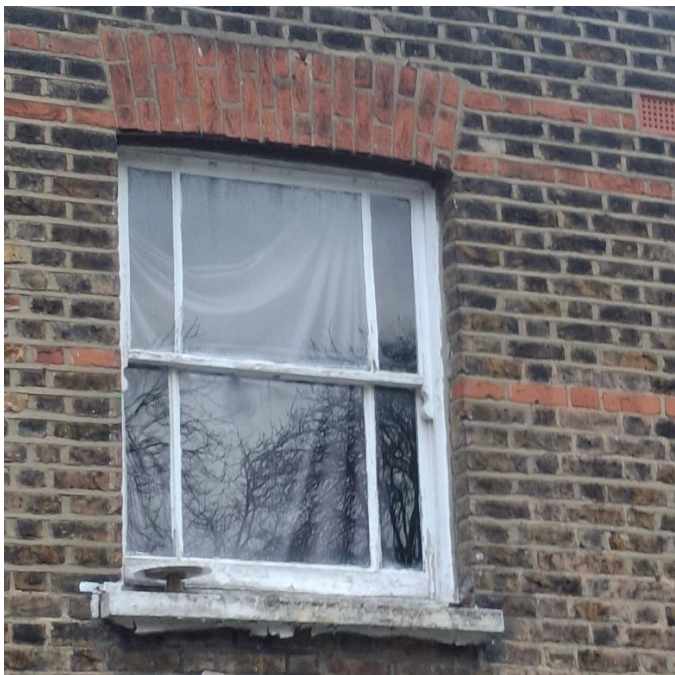
Rear Addition 1 st Floor Sash Window
