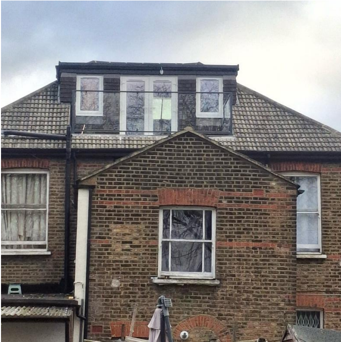
Rear Addition 1 st Floor Sash window with UPVC dormer roof structure
