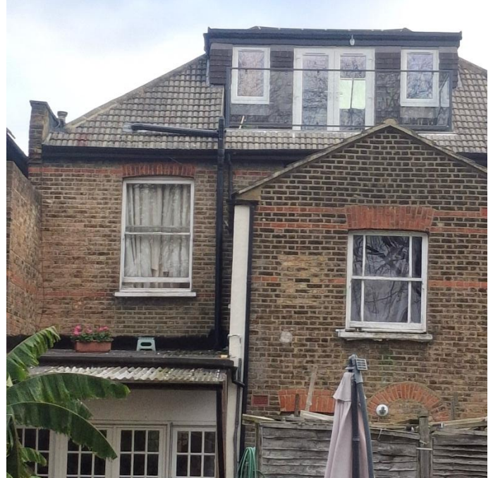
Rear Elevation 1 st Floor Sash window with UPVC dormer roof structure
