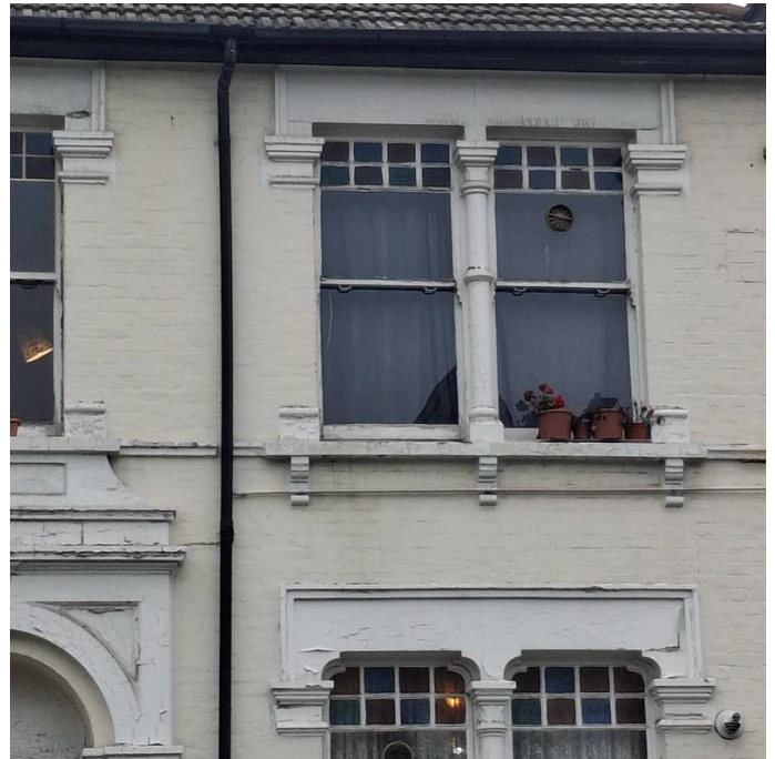
Front Elevation 1 st Floor Sash Windows
