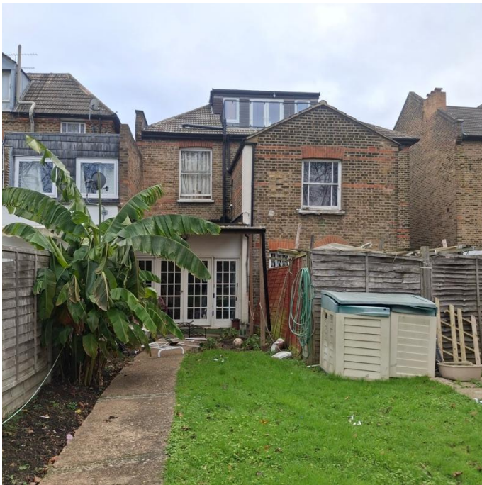
Rear Elevation windows
