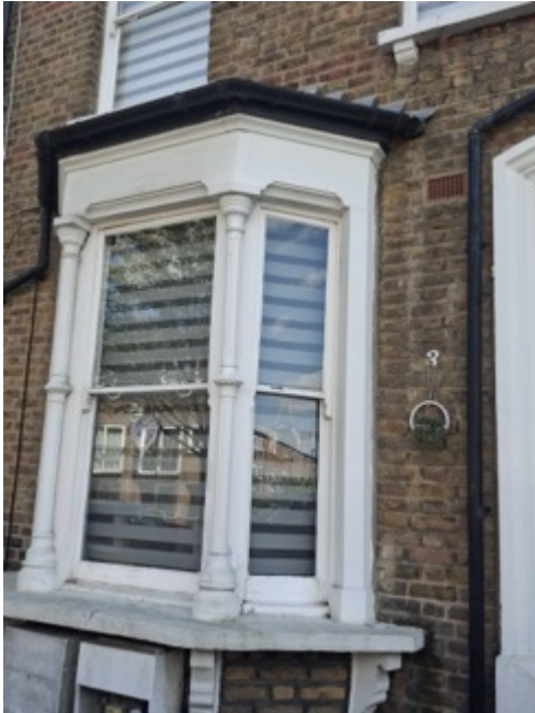
Front Ground Floor Bay Window
