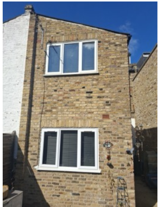
Rear End Ground & First Floor Windows
