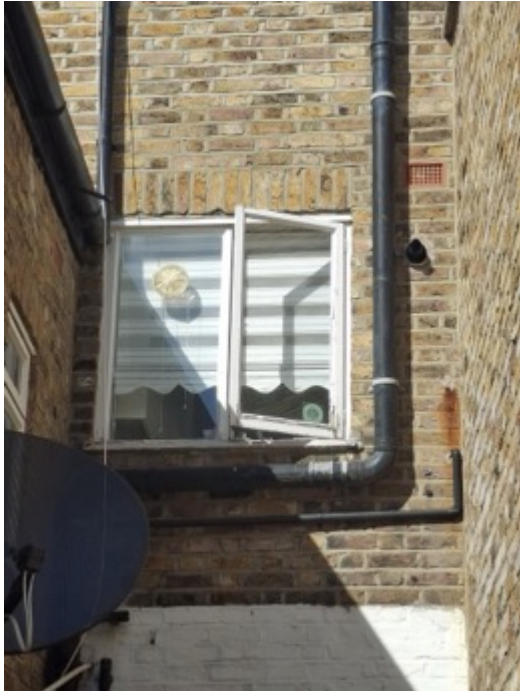
Rear First Floor Window
