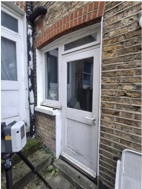
Rear Side Exit Door
