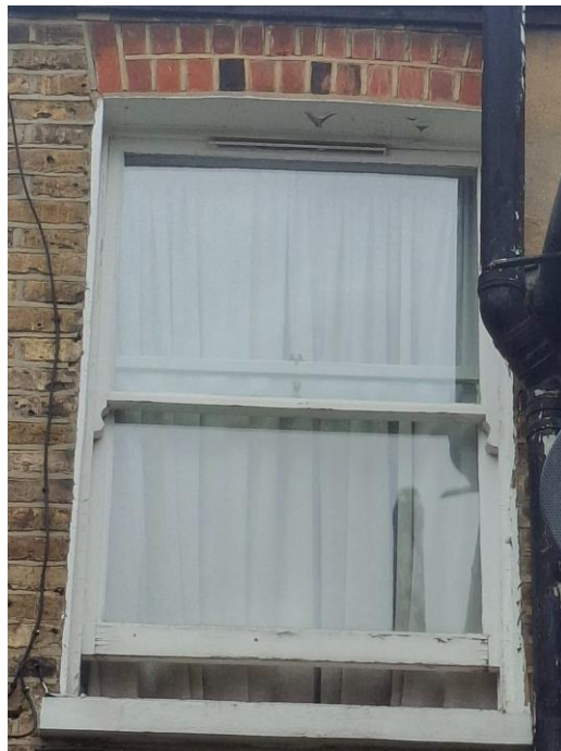
Rear First Floor Window
