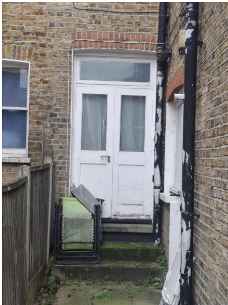
Rear Exit Door
