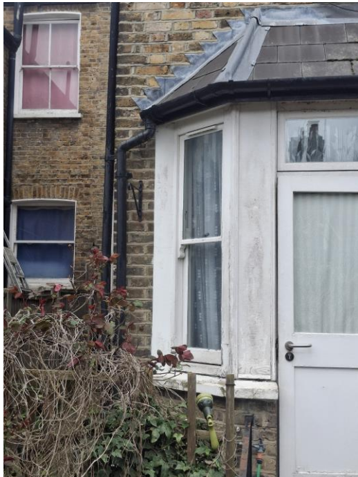
Rear End Ground Floor Window
