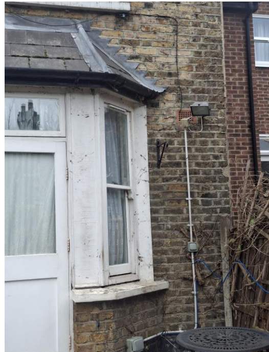
Rear End Ground Floor Window
