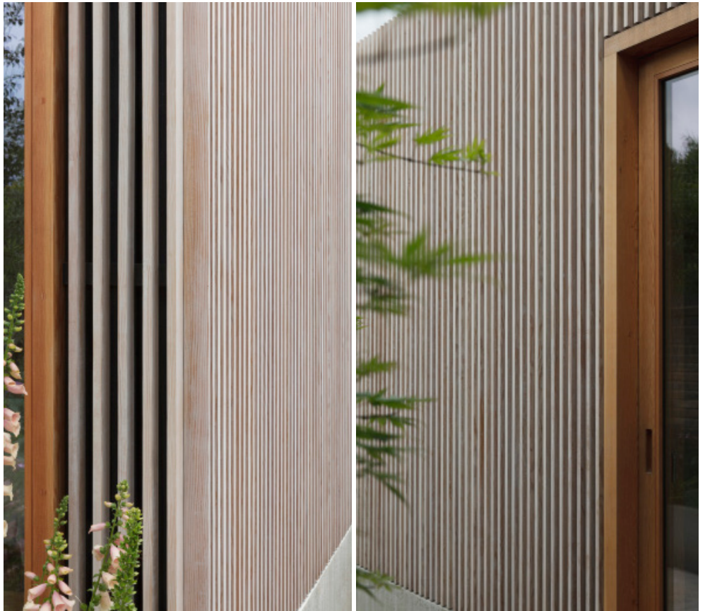
High quality Douglas Fir cladding with open joints and bespoke profile. Planed-all-round square edge profile 50x25mm section sizes in an oiled finish.
