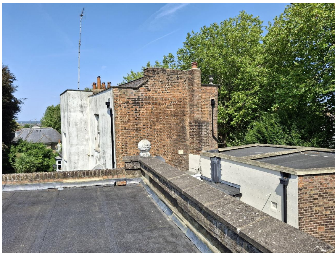
Figure 7. The rear of Number 47 And 49, North Hill as seen from the subject property
