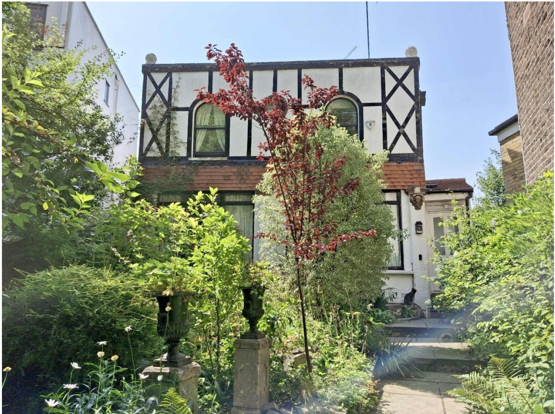
Plate 1. The subject building as seen from inside the brick boundary wall, facing west
