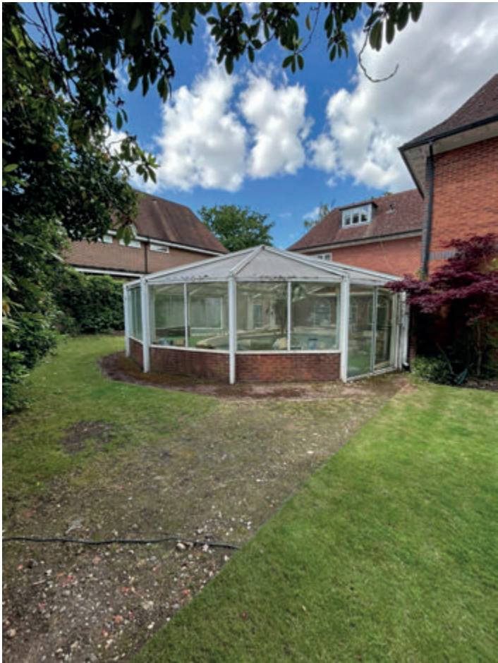
Fig 6. View Park House existing swimming pool extension
