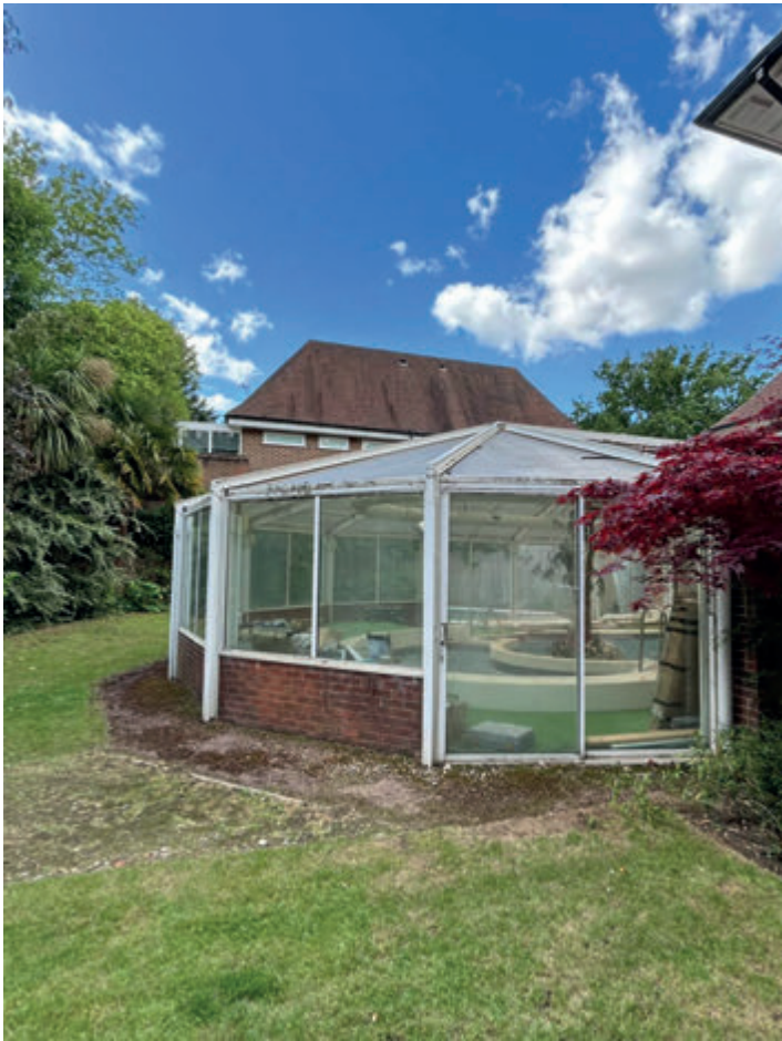
Fig 7. View Park House existing swimming pool extension, Red House in background
