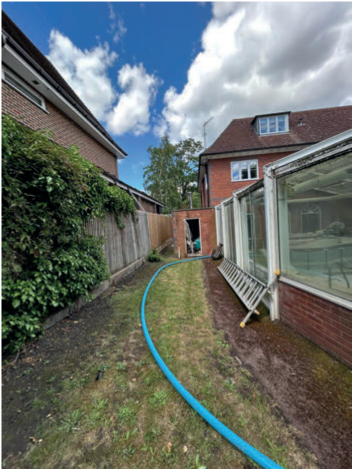
Fig 4. View towards rear between Red House and Park House
