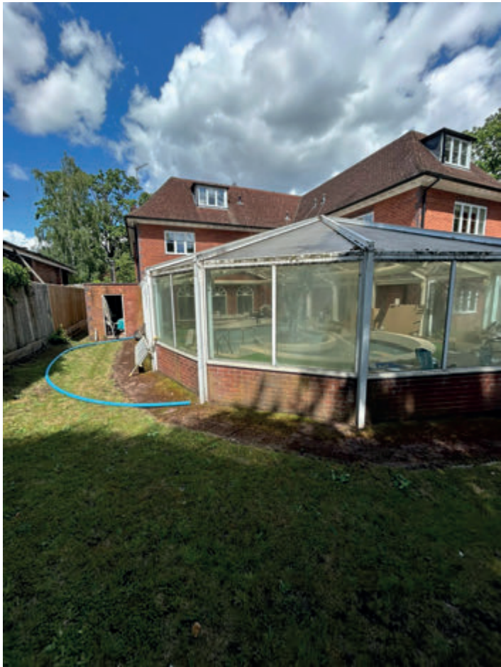
Fig 5. View Park House existing swimming pool extension
