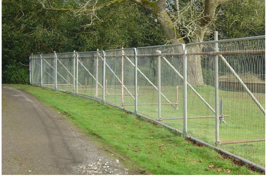
Fig.1: Weld-mesh tree protection fencing (blue line) Purpose: To create an exclusion zone around exposed areas of the RPA. Fencing shall prevent all construction access. Specification shall be as follows: 1) Scaffold framework 2) Heras or similar weld mesh panels 3m x 1.8m or similar approved, bound to framework with cable ties 3) Anti-tamper couplers between panels min. 1m apart and 2 per panel join 4) Ground level - fencing shall not allow gaps for access 5) Supporting struts to be impact resistant wherever possible
