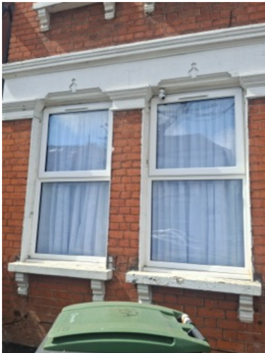
Front Ground Floor Windows
