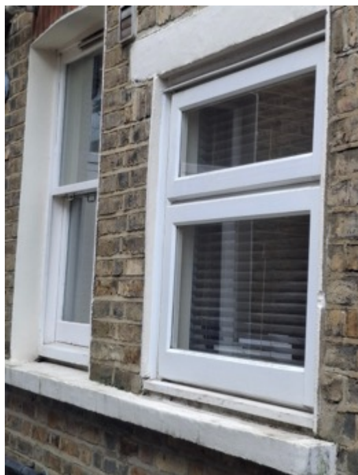
Rear Side Ground Floor Windows
