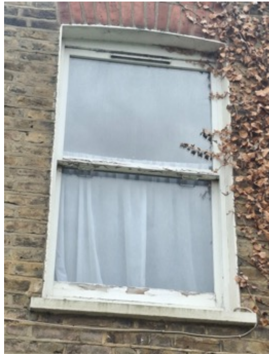
Rear End First Floor Window
