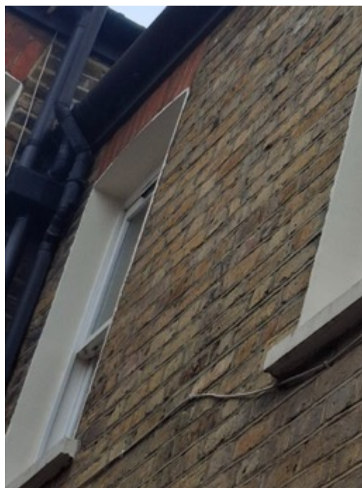
Rear Side First Floor Window
