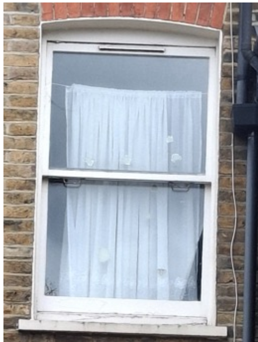
Rear First Floor Window
