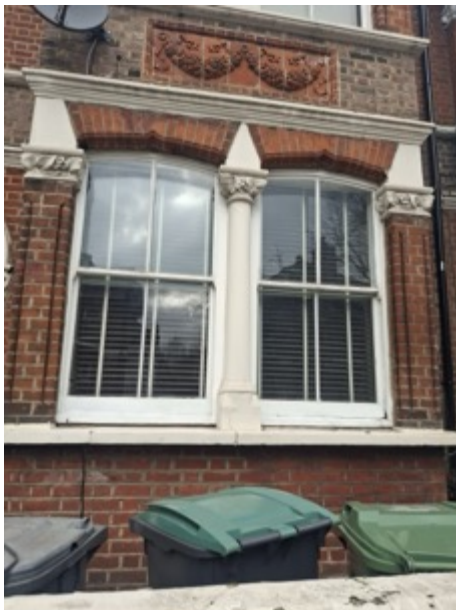
Front Ground Floor Bay Window
