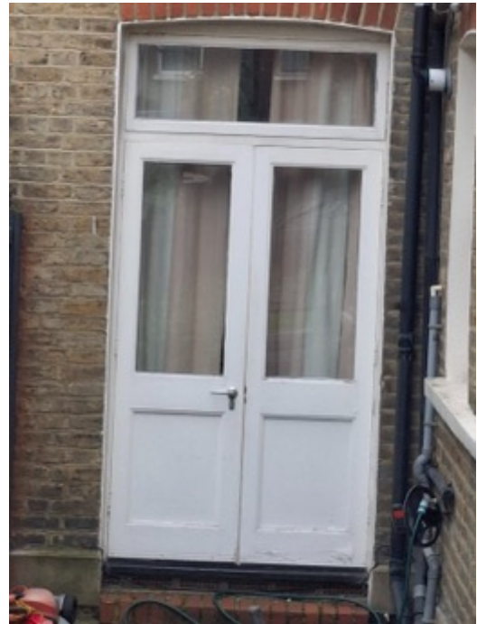
Rear Patio Exit Door
