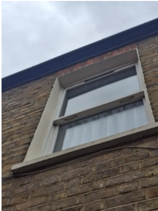
Rear Side First Floor Window
