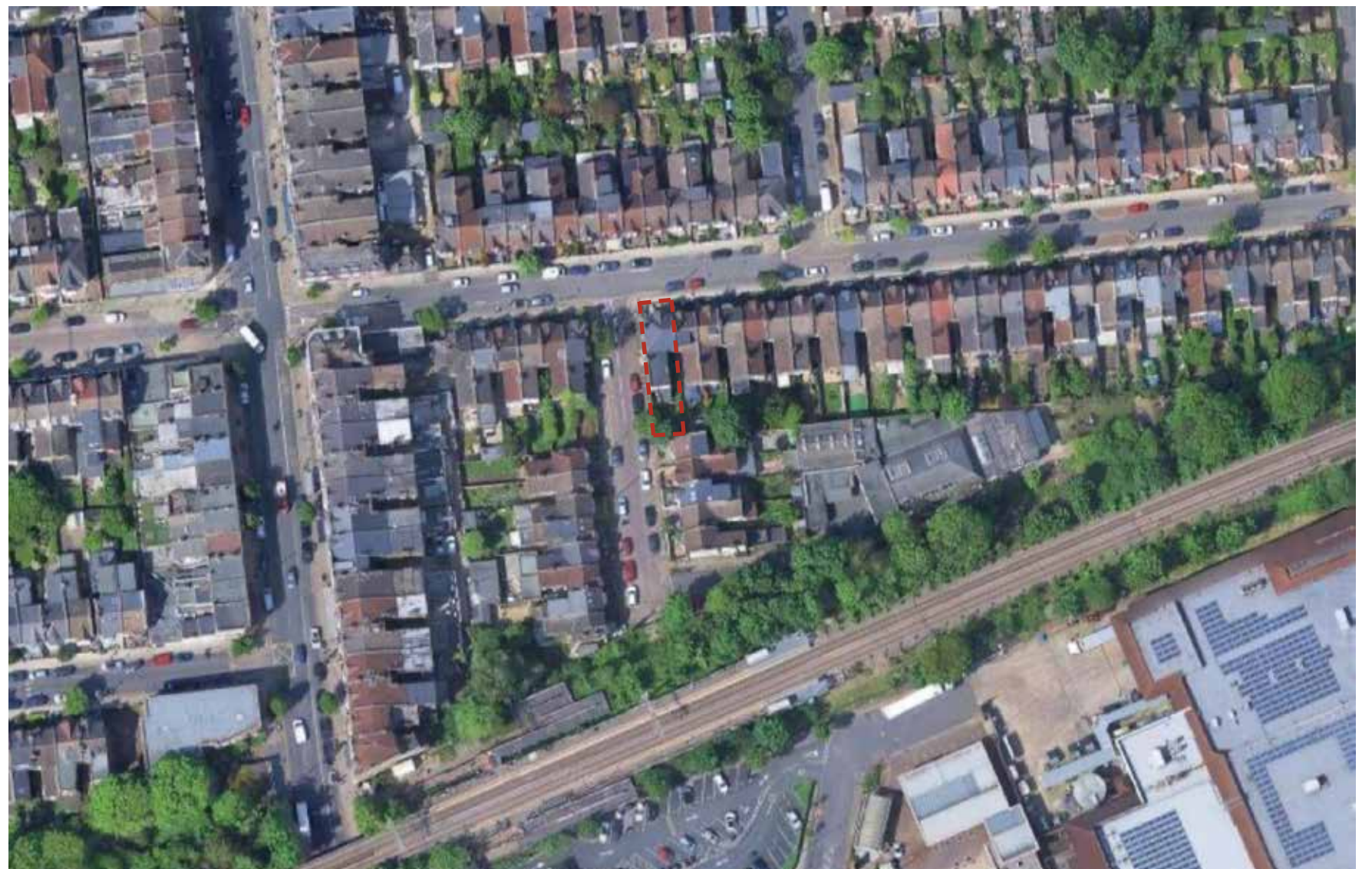
Aerial image of existing site and context (Not to Scale)
