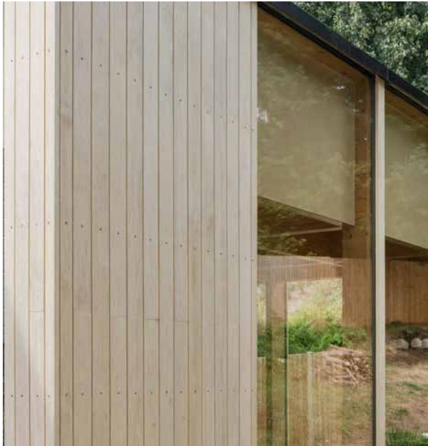
GF REAR EXTENSION & DORMA ACCOYA CLADDING
