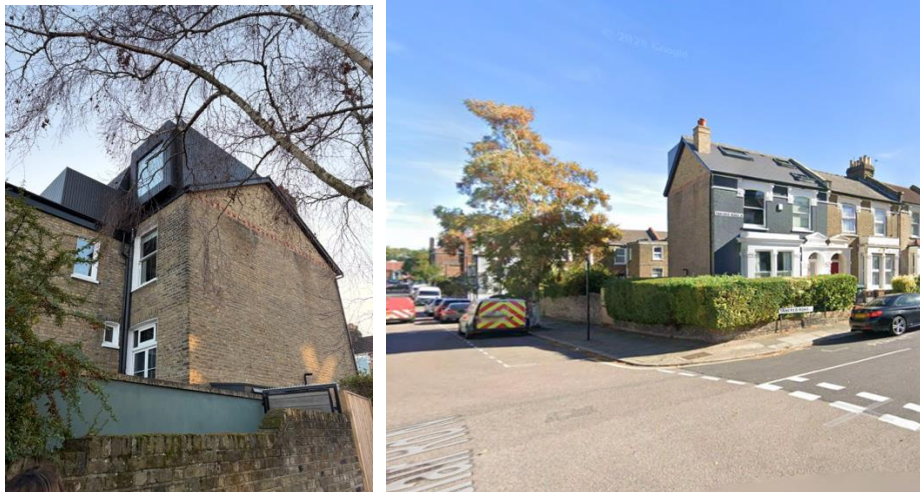
Fig. 6 Hip-to-gable and rear dormer extension from no. 12 Tancred Road (HGY/2021/1611).
