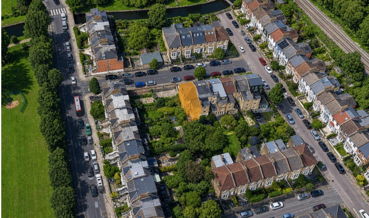
Fig. 1. Aerial view of 2 Tancred Road and the immediate surrounding context. The building is highlighted in orange. June 2026.
