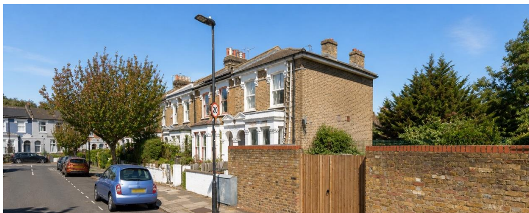
Fig. 3. Existing side context of 2 Tancred Road, showing the south view of the house.
