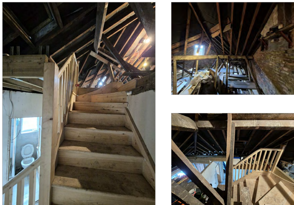
EXISTING ATTIC & STAIRCASE
