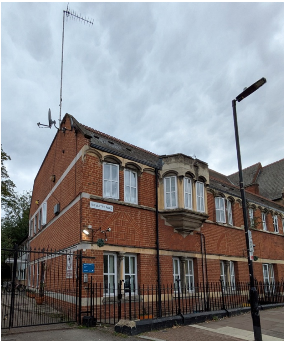
Image 1 Front Elevation of 188 Vartry Road
