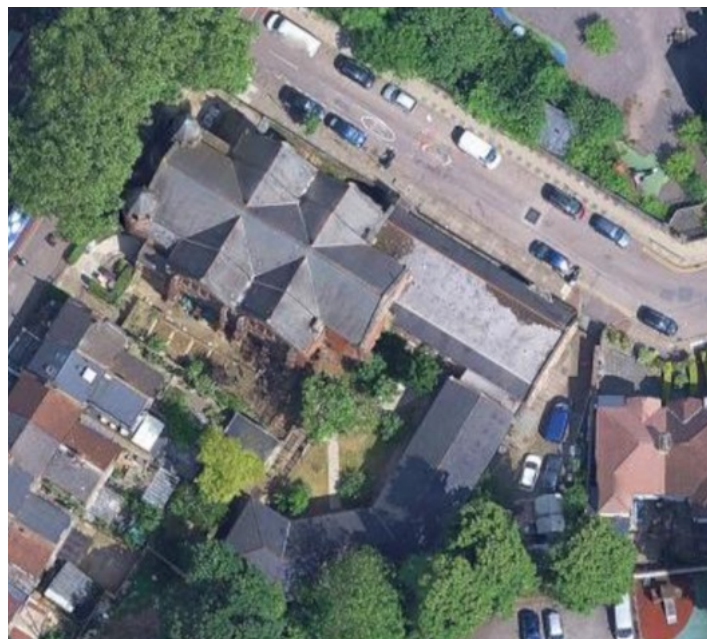
Image 10 Aerial view of existing roof
