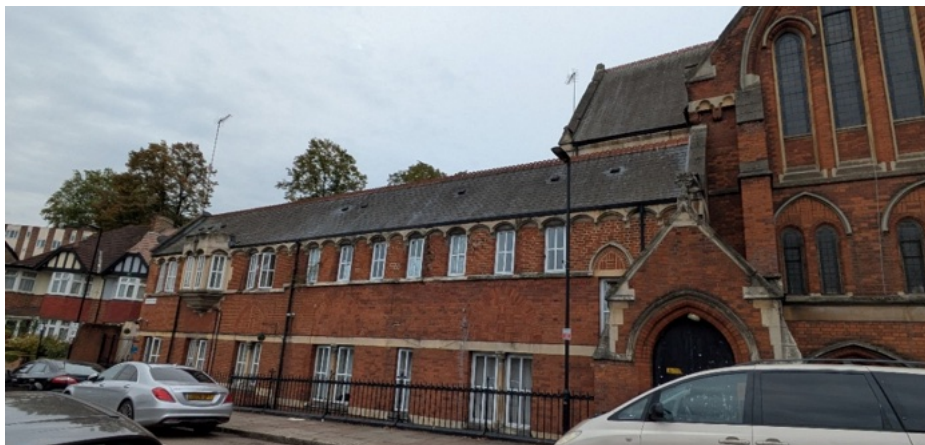
Image 6 Front Elevation with Woodberry Down Baptist Church
