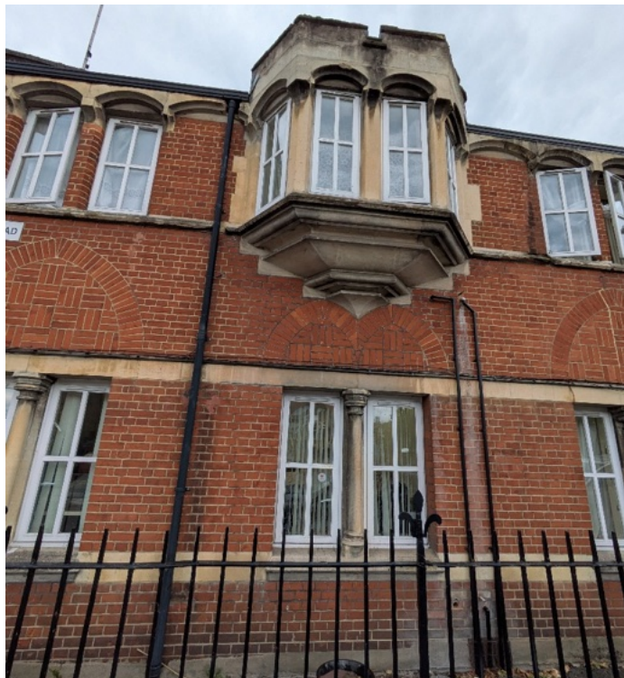
Image 7 Significant architectural features to the Front Façade
