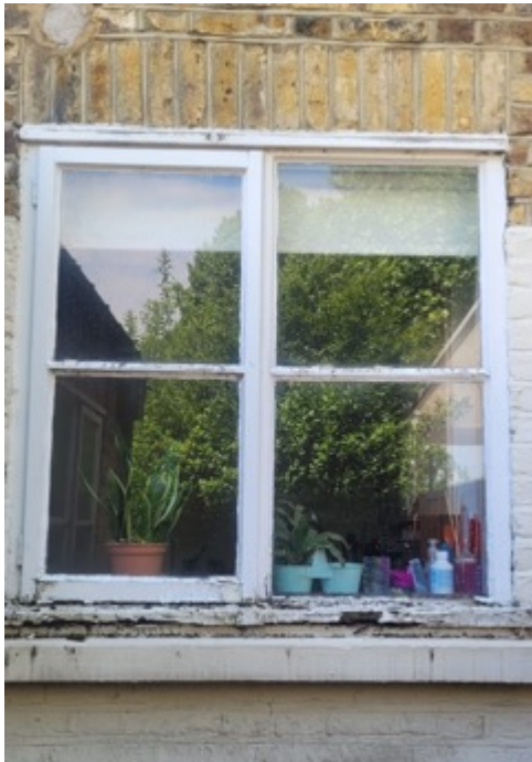
Rear Ground Floor Window
