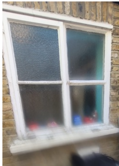
Rear Side Ground Floor Window
