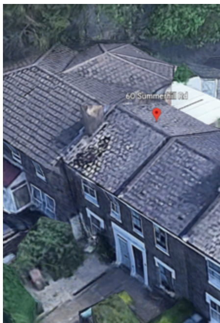
Roof Side Elevation (South)
