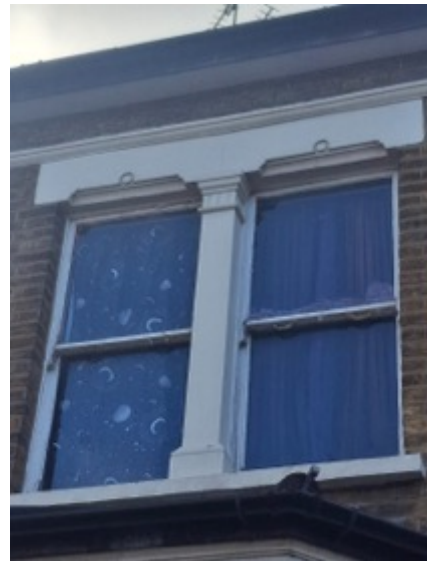
Front First Floor Windows
