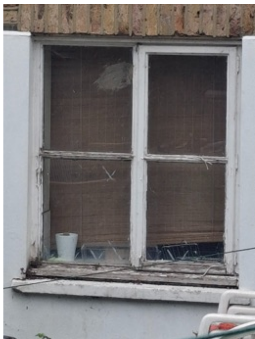
Rear End Ground Floor Window
